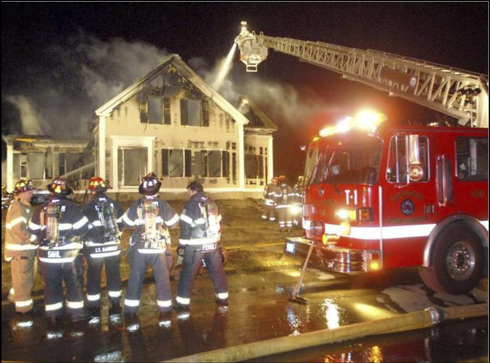
November 24, 2010: An arsonist burned a $500,000 home still under construction at 16 Boulder Brook Road in Sandwich, MA.
