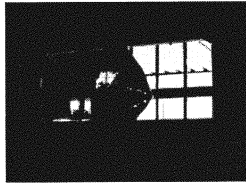
Broken glass in cell window. Hopi, AZ
