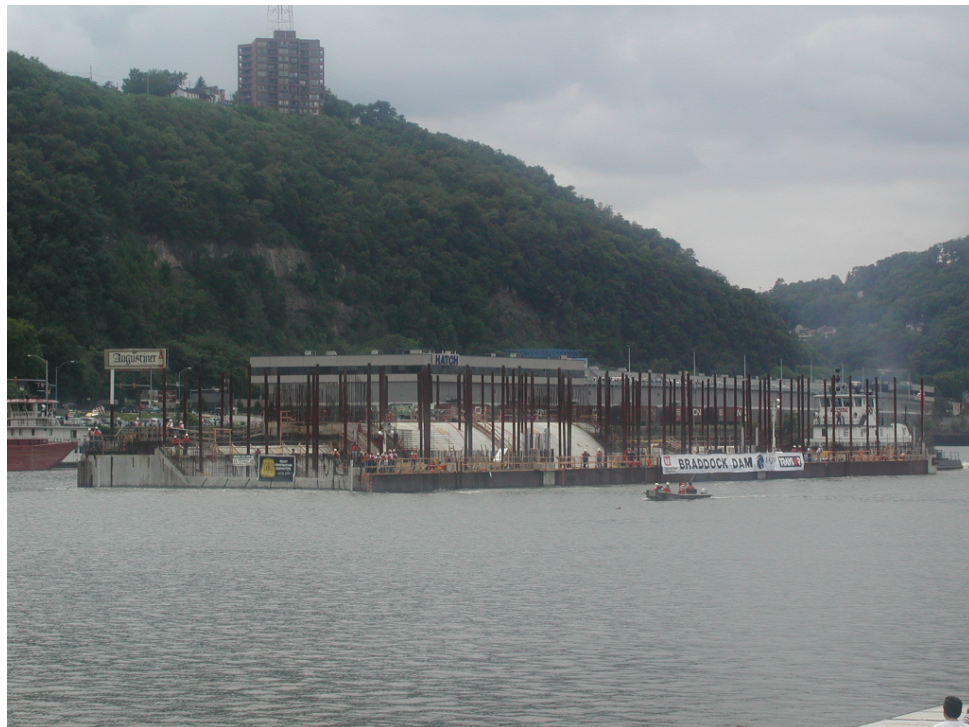
Figure 3 - Braddock Dam being floated up the Monongahela River on July 26, 2001
